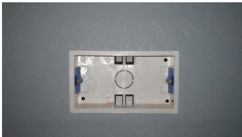
Figure 3 Switch box before installation of Putty Pad
