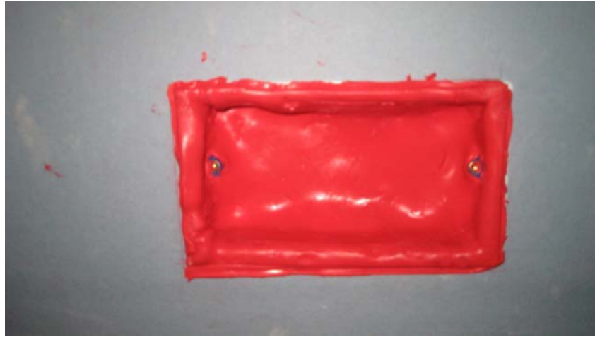
Figure 4 Putty Pad installed inside switch box
